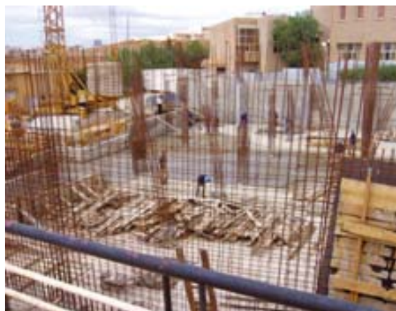
Figure 3: View onto the building site of the clean room.
