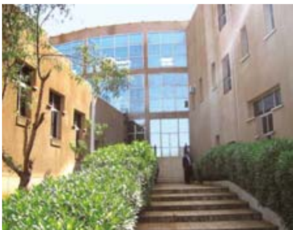
Figure 2: Entrance of the in the year 1988 founded institute.
