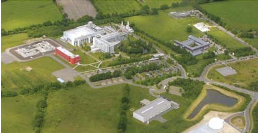
High Tech Itzehoe: SMI (red building), Fraunhofer ISIT and Vishay Siliconix Itzehoe (largest complex) Bullith Batteries and Condias (bottom), IZET Innovationszentrum (right), Nippon Antenna (white round building) and Procon (upper right).
