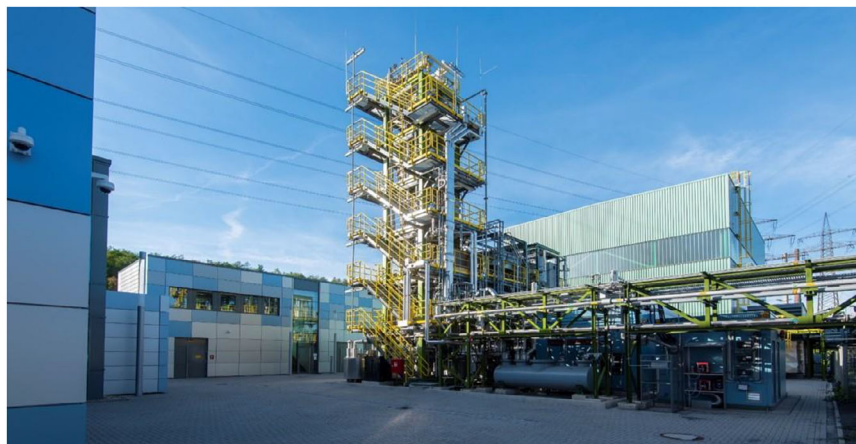
FIGURE 1 | View of the Carbon2Chem technical center in Duisburg.
