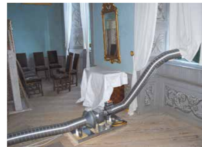
Experimental setup for indoor climate control using adaptive ventilation at Skokloster Castle, Sweden (Figure 2b)
