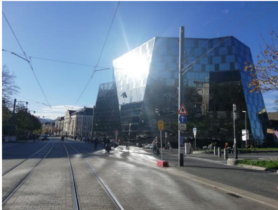
Figure 8: Example for a glare situation (new library of the university of Freiburg); image is courtesy of Fraunhofer ISE, taken from the website bipv-bw.de
