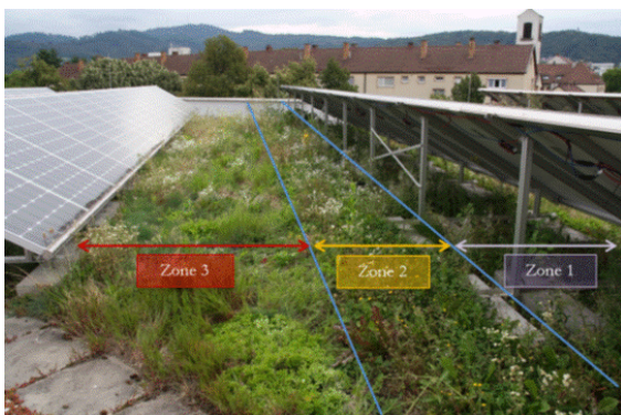
Fig. 1 Three zones of vegetation, modules close to ground shown at an existing non-APV site.
