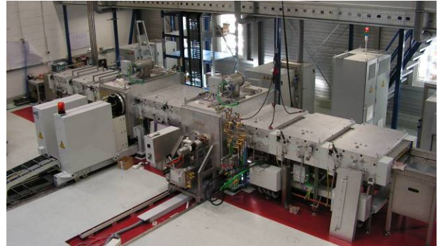
Figure 1: Picture of the ATON 500 based evaporation equipment.
