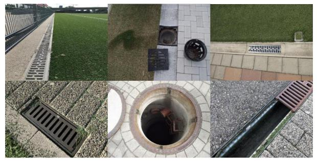
Figure 6: Different drainage elements: Drainage channel bordering the pitch, trough channel with gully shaft, trough channel with grating shaft, open drainage channel, open dry well, smaller grating shaft (from top left counterclockwise).
