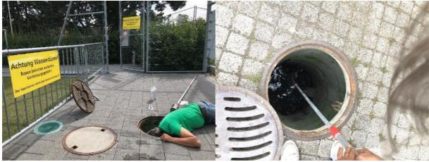
Figure 50: Assessment of inspection shaft (I.); taking of a water sample from the inspection shaft (r.)
