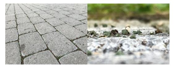
Figure 27: Infill next to the pitch on paved and unpaved surfaces
