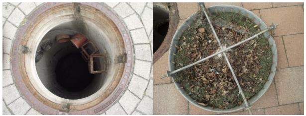
Figure 49: Dry well with drainage outlets (I.); strainer with retained performance infill (r.)
