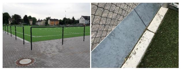
Figure 4: Paving around an artificial turf pitch (I.), surrounding metal strip to retain infill (r.)
