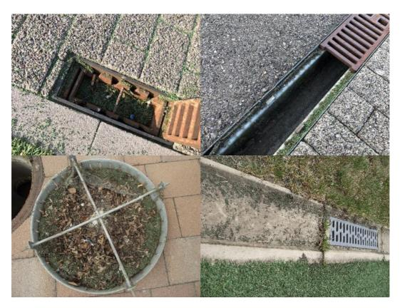
Figure 26: Rubber granulate in drains and channels
