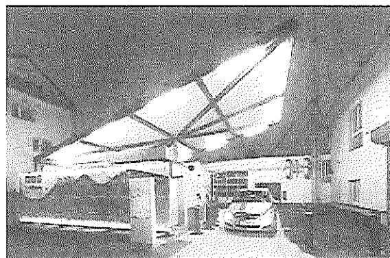
Fig.2 Freiburg solar hydrogen filling station at Fraunhofer ISE. Photovoltaic modules generate power and a PEM electrolyser and produces hydrogen at 30 bar. The hydrogen then is compressed and pre-cooled so that the dispenser operates according to the SAE J2601 protocol. Slow fill at 350 bar is possible. The filling station is approved by German CEP.
