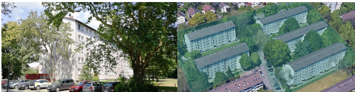
Figure 1: Photo of the building (left, © Stefan Hess, INATECH ) and the district (right, © Google Earth, Map data: Google, GeoBasis-DE/BKG)
