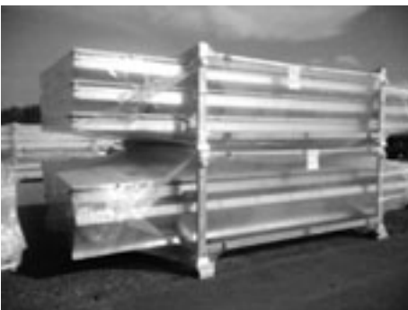
Figure 3: two bundled crates with facade elements in the field storage [3]
