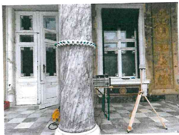
Figure 1: the new system on a column of the Marmorpalais in Potsdam.
