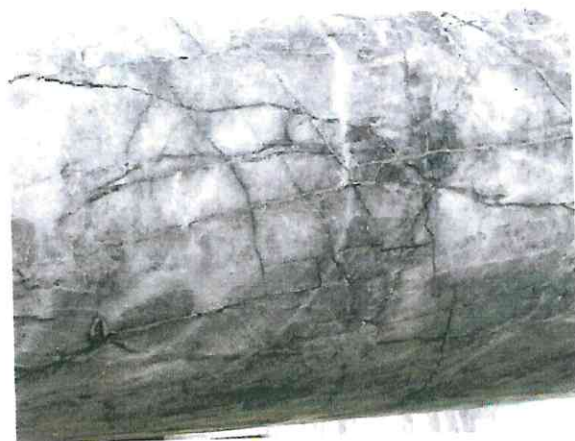
Figure 5: typical structure of the marble columns of the Marmorpalais in Potsdam.
