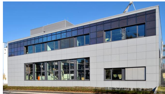
Figure 5: Façade application of 70 TPedge BiPV modules at Fraunhofer ISE, Freiburg
