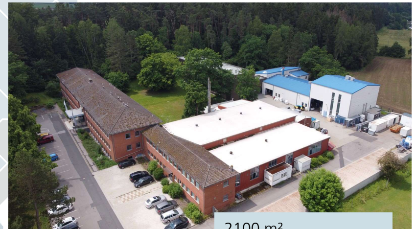
2100 m 2 Technical Center
