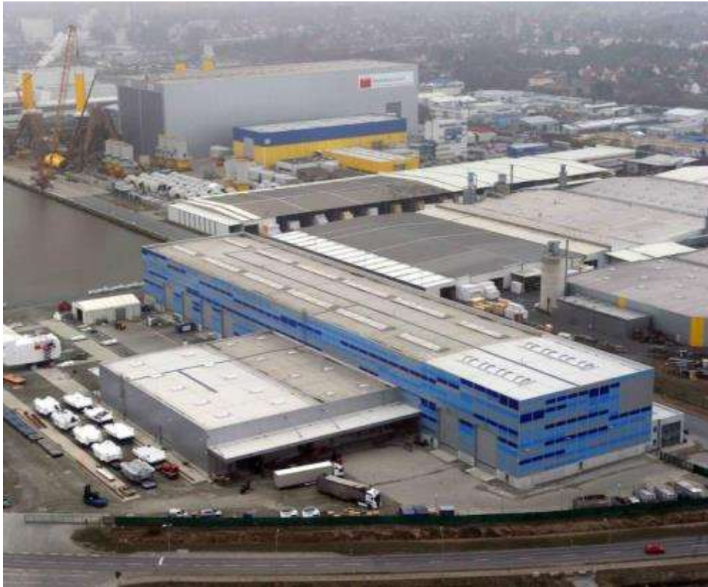
Senvion production hall for assembly of large nacelles and hubs
