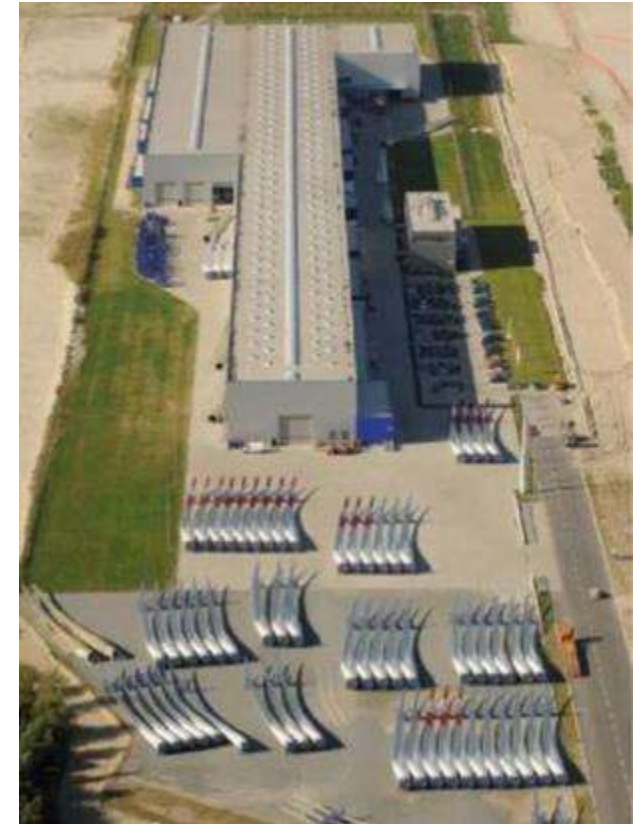
PowerBlades factory for Offshore blades
