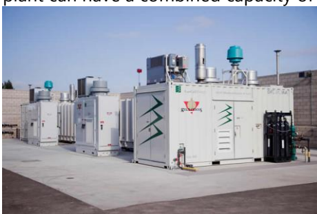
Photo: Many fuel cells, like these FuelCell Energy units, can run on natural gas or biogas
