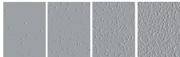
Figure 6. Alterations in a surface due to the effect of chemicals over a period of time (from left to right)
