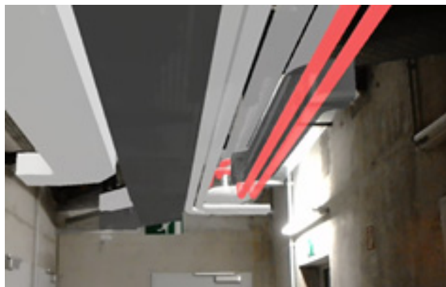
Fig. 7. MR use case for visual comparison between BIM model and realization of the MEP system
