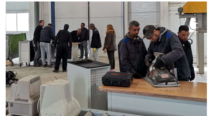
Installation of e-waste treatment plant in Tunis
